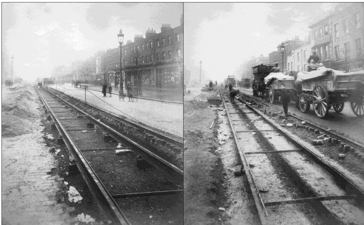
Rails in position in the Mile End Road opposite the Paragon, ( left ) and track ready to receive conduit pipe opposite the Anchor brewery. ( right )
