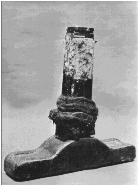
A Griffiths-Bedell stud, probably one removed from Bow Depot in 1939 at the time it was being converted for trolleybuses.
