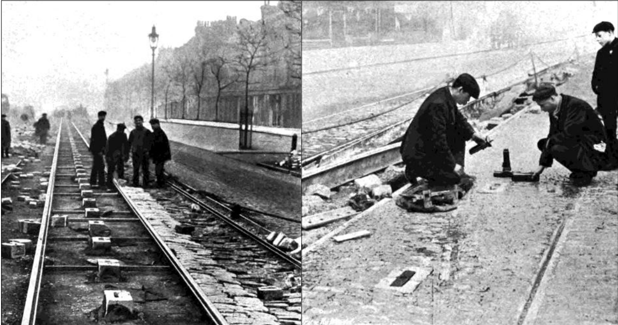
In the Mile End Road with the granite boxes ready to receive studs, ( left ) and with the road surface made up, the studs are actually being. ( right )
