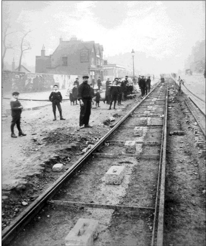
Track with granite blocks ready for receiving studs near Mile End Station
