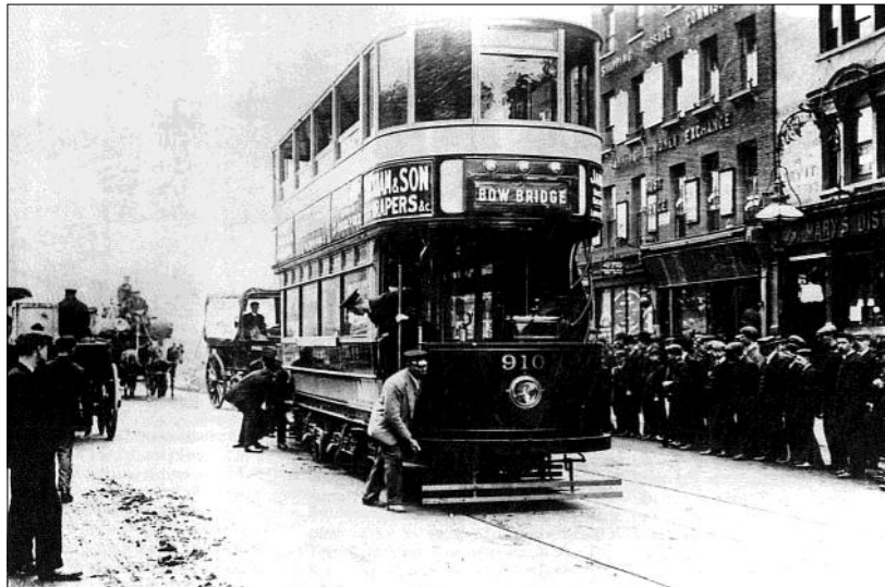
The interested crowds watch a stuck L.C.C. E/1 910 being manually pushed onto the next live stud in July 1908 during the ill fated trial. Note also the typically large amount of muck in the road to the bottom left of the view.
