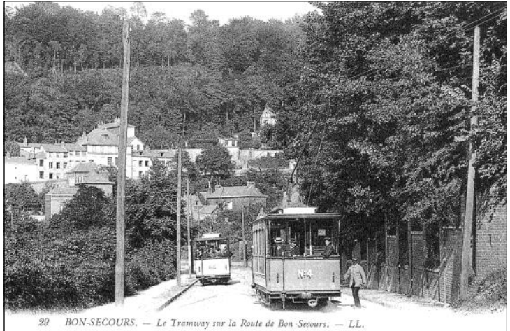
Cars 2 and 4 at the on-street passing loop at Grâce de Dieu
