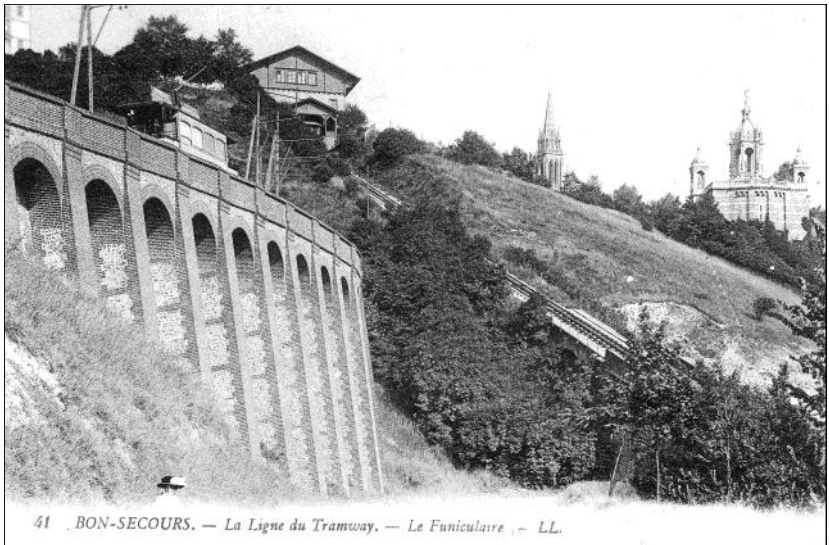
On the left is the tram viaduct, in the centre the funicular track and on the right the Basilica of Notre-Dame de Bonsecours.
