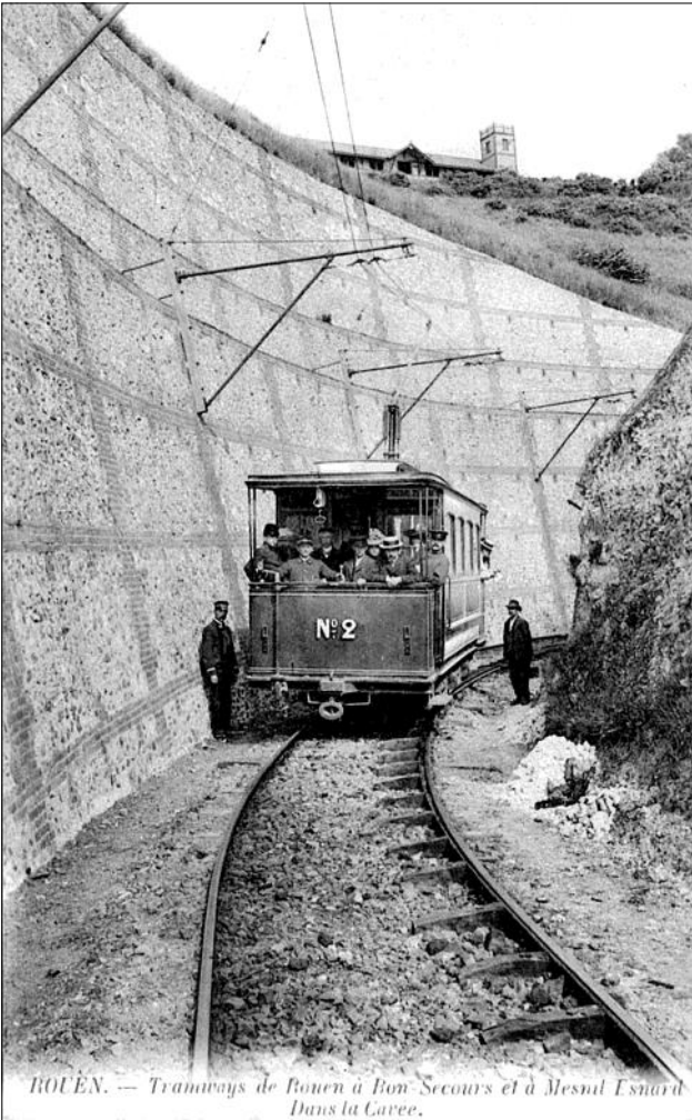
Car 2 in the cutting as the tram leaves the horseshoe loopback and proceeds up the incline towards Bonsecours. Note the fixings for the check rail.
